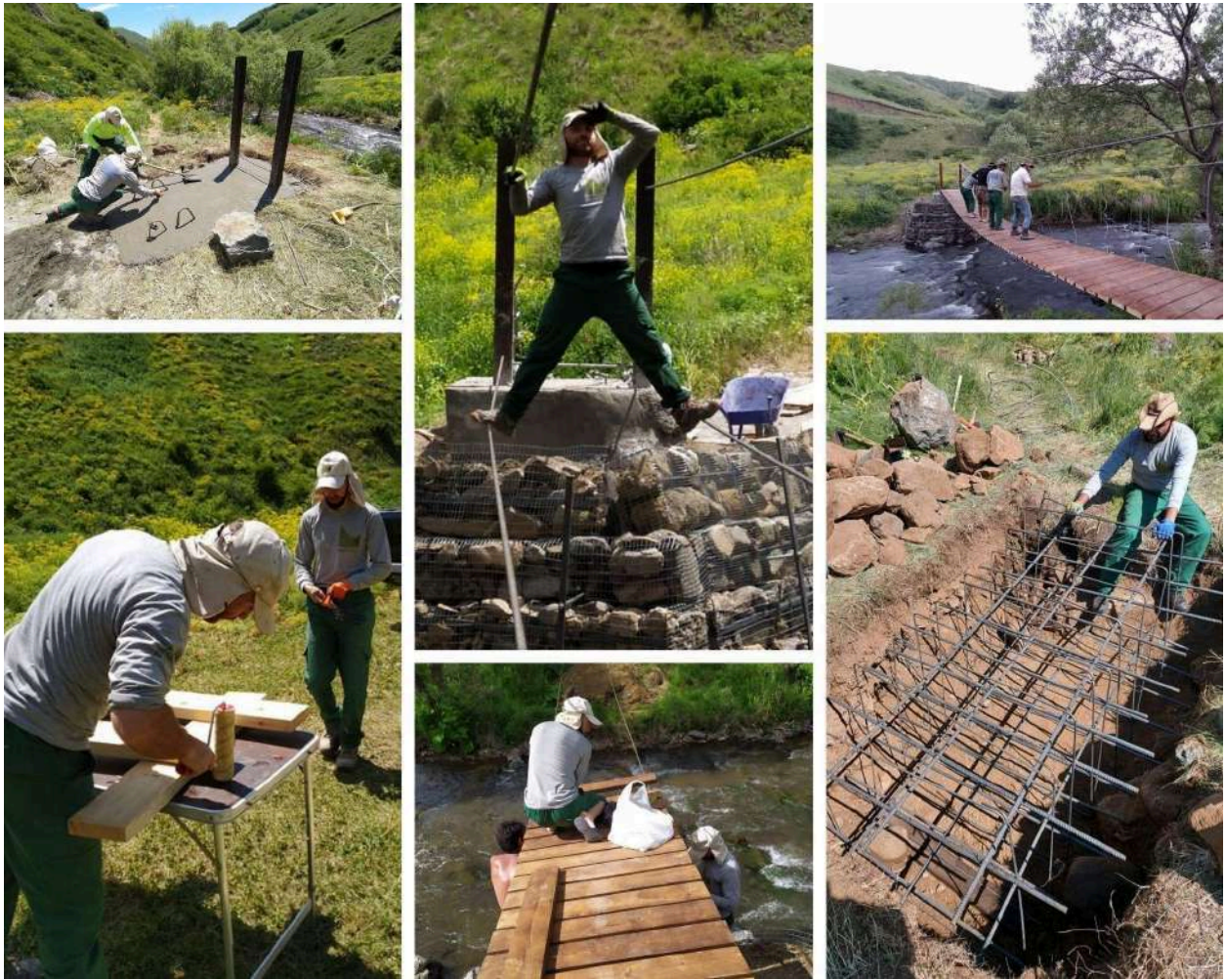
Photo #1: Trchkan bridge construction process
